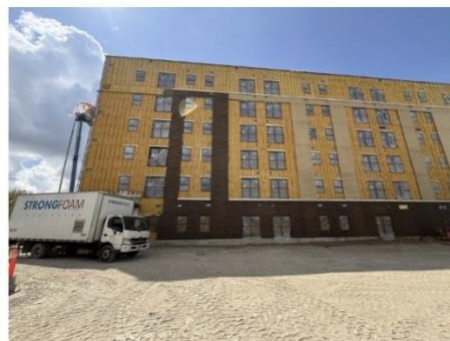
Partial view of North Elevation.
